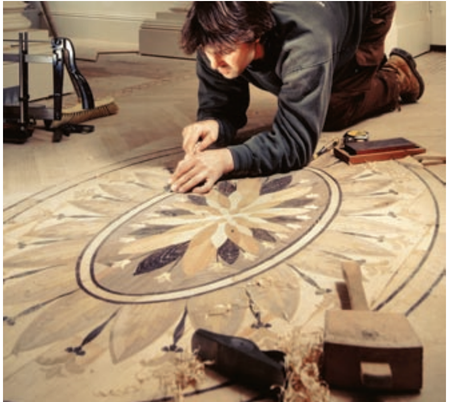
Figure 8: A Weldon craftsman working on a new decorative panel in wenge, teak, walnut and oak at Regents Park, London.
